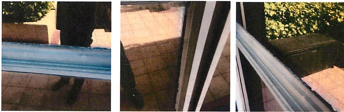
Figure F: Exterior sealant at window frame that has aged past its serviceable lifespan
